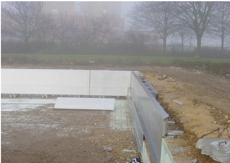
The stainless steel elements are directly mounted on the stripped wall
