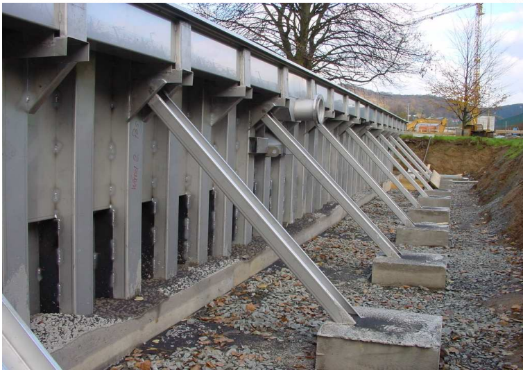
The rear support supports the stainless steel walls
