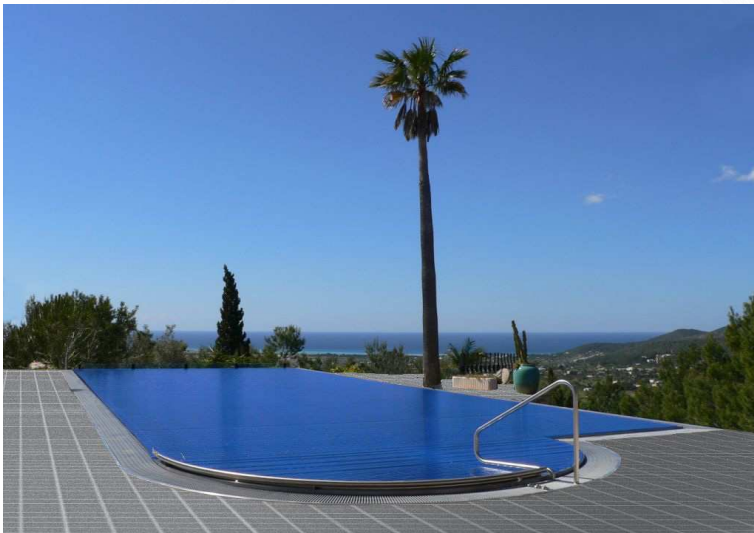
Rehabilitated pool with a lamella cover and glass face wall Water surface: 94.5 m² | Year of construction 2005
